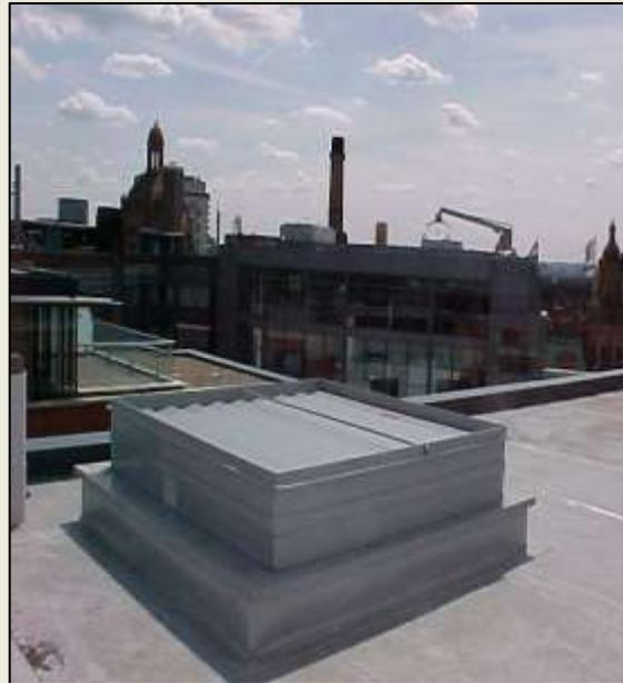
**Figure 14(b)** Roof mounted Automatic opening vent
