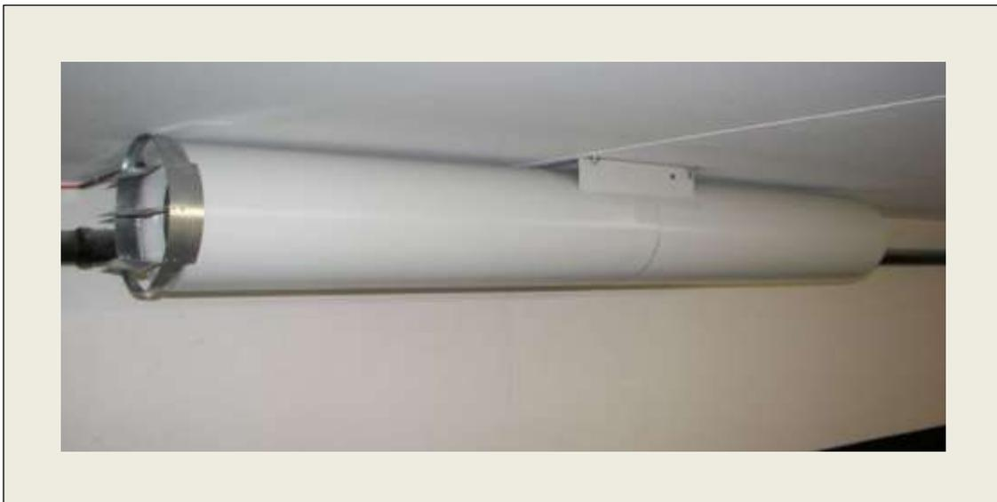
**Figure 16** Car Park impulse Ventilation Fan
