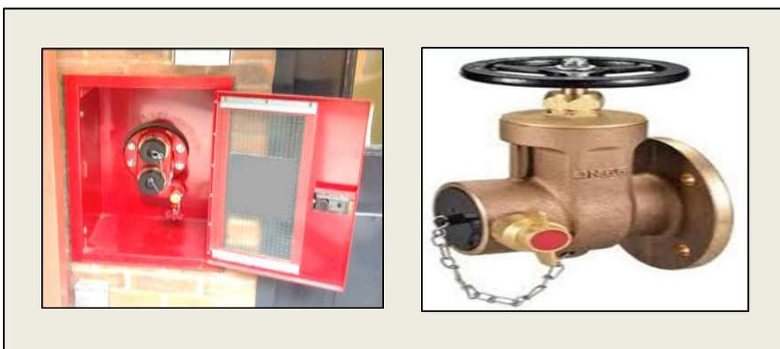
**Figure 11(a)** Inlet Breeching at exterior of building
